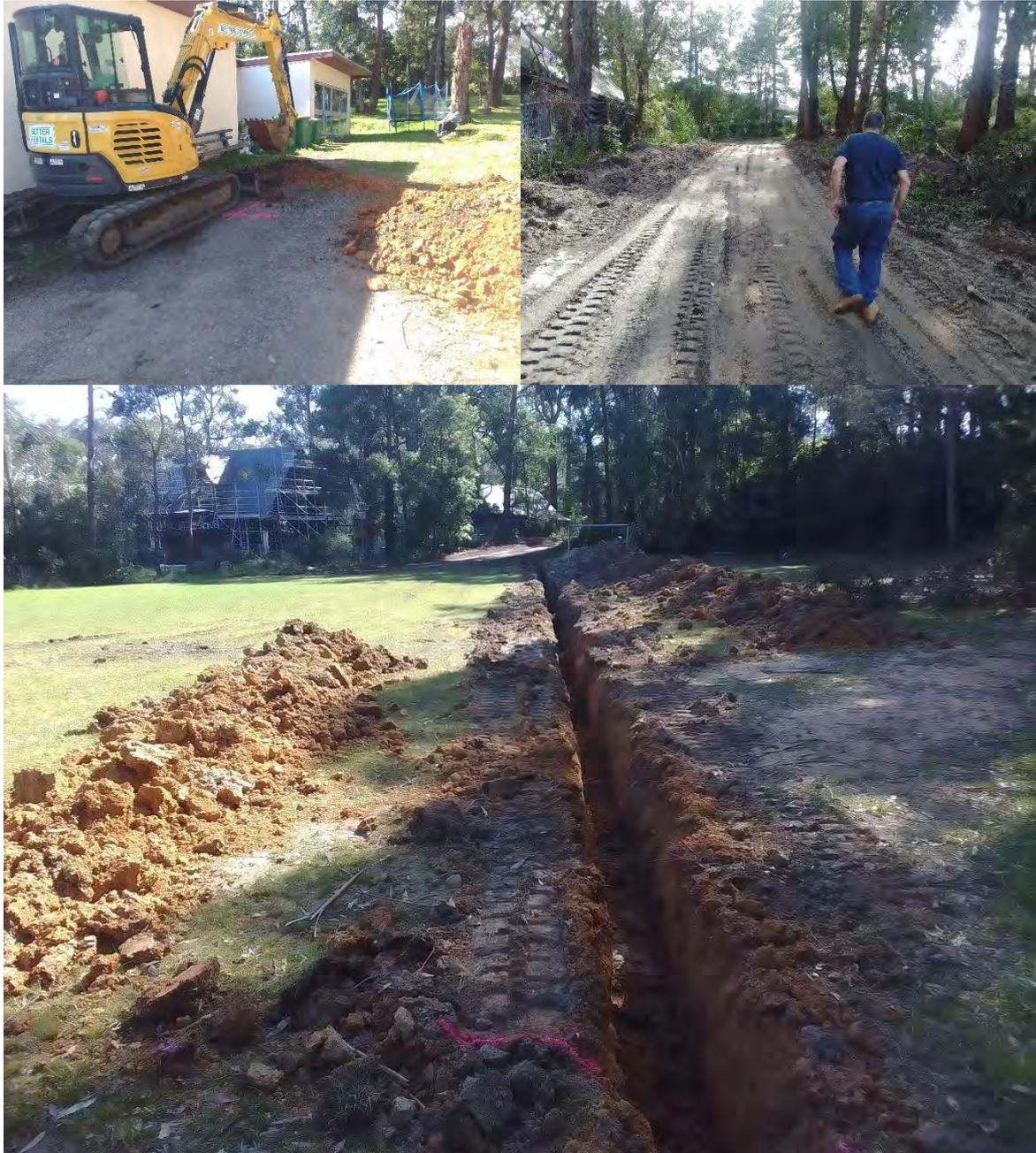
James Babb and Chris Bruce have been working hard, developing the lower driveway entrance to the Belgrave property and digging trenches for the Sewerage, grease traps and electricity. The project should be completed by the end of October.
