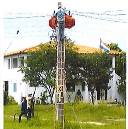
**An ANDE engineer from Olimpo is installing a new fuse.**
